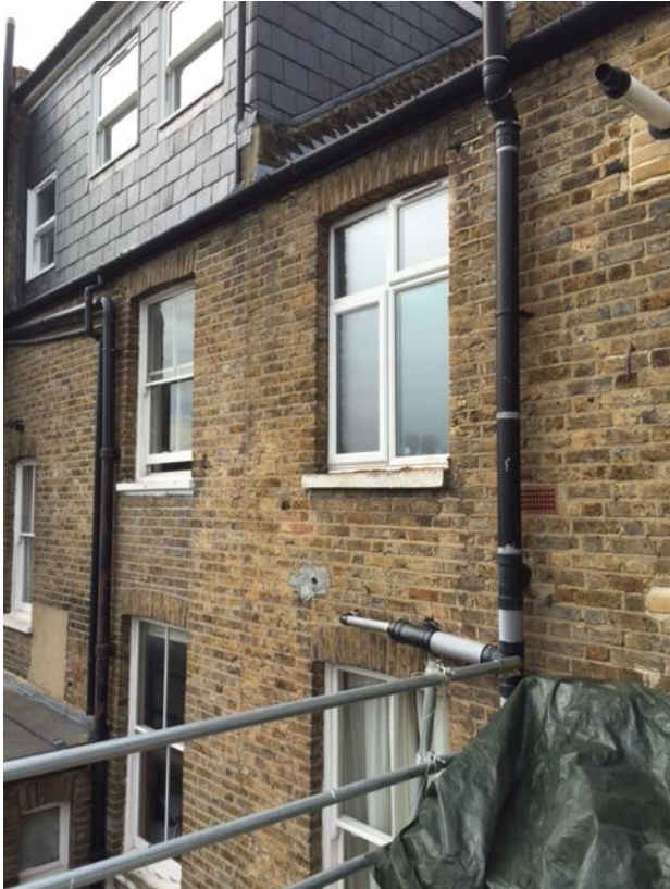
Image 6 – View towards no. 62 Beversbrook Road
