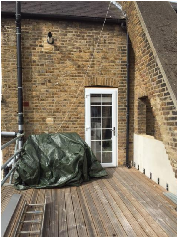
Image 3. – View of existing flat roof
