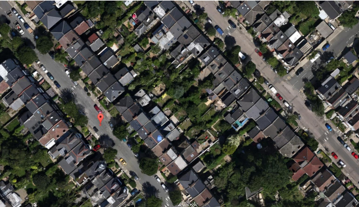
Image 1. Aerial view of the site
